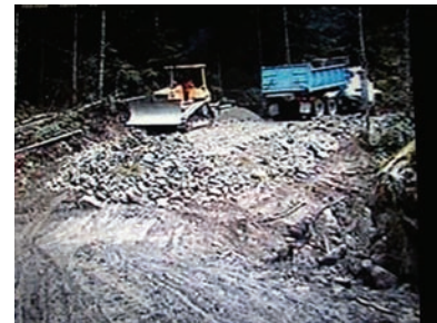
RALMAX GANG HARD AT WORK – FILLING AND SHAPING THE ACCESS ROAD
